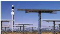
Solar tracking systems for a power plant in the U.S.
